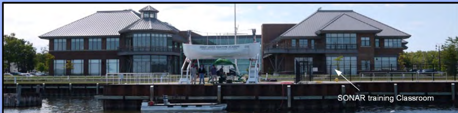
Northwestern Michigan College Training Facility
